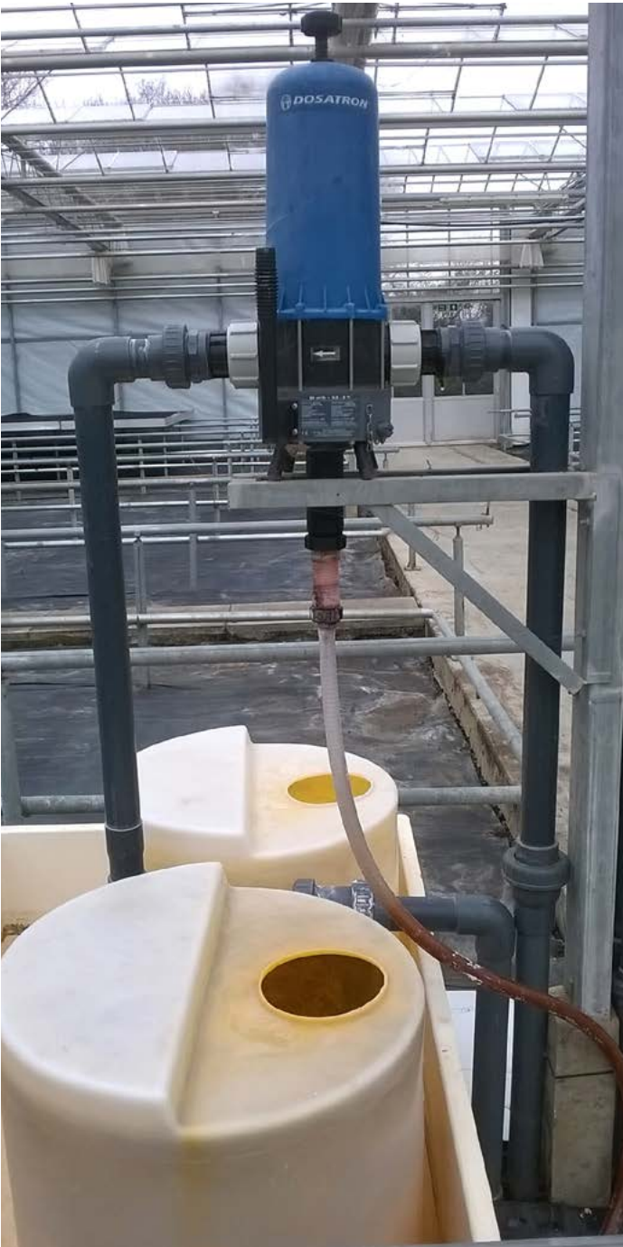
Figure 6. Typical water-powered proportional dilutor used for the application of water soluble fertilisers to crops
