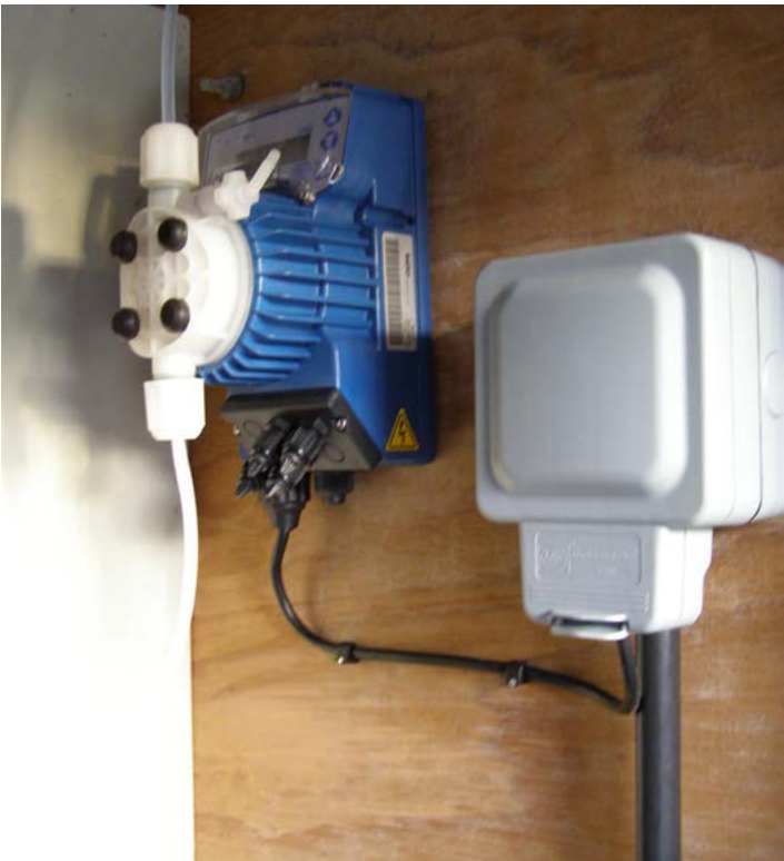
Figure 9. Automatic acid dosing equipment and acid storage to adjust irrigation water alkalinity
